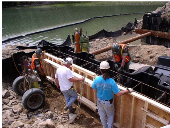
Navy Seabees construct the new bridge
