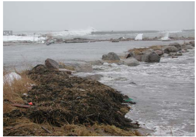
Seawater breaches the barrier beach flooding into the marsh during a winter storm
