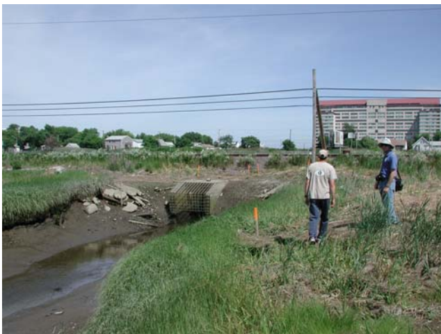
Project partners survey the existing culvert
