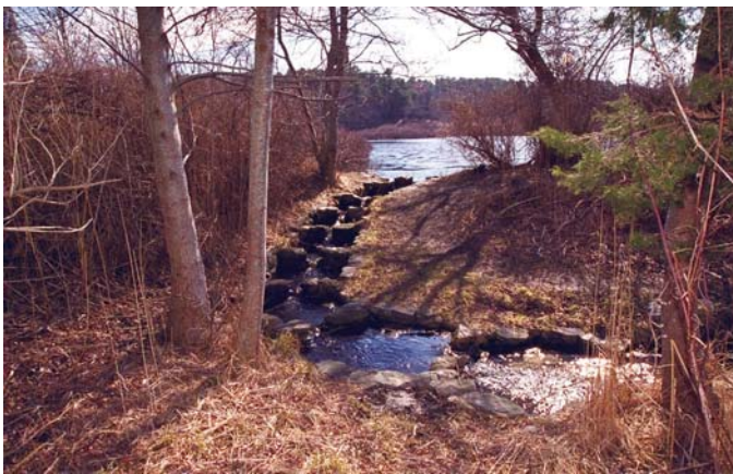
A fish ladder aids alewives in their upstream migration on Quivett Creek
