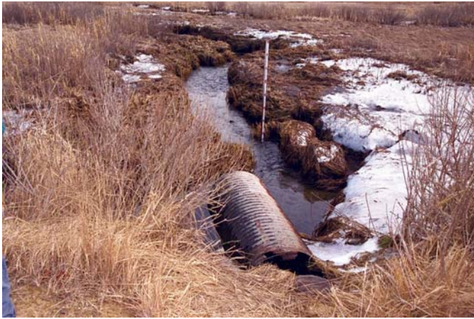
One of the existing culverts at Quivett Creek
