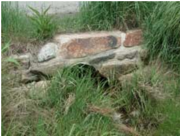
Existing culvert under Seaview Street
