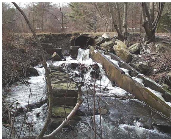
Billington Street Dam and Fishway
