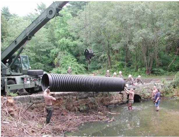
US Army Reserves help to remove the Billington Street Dam
