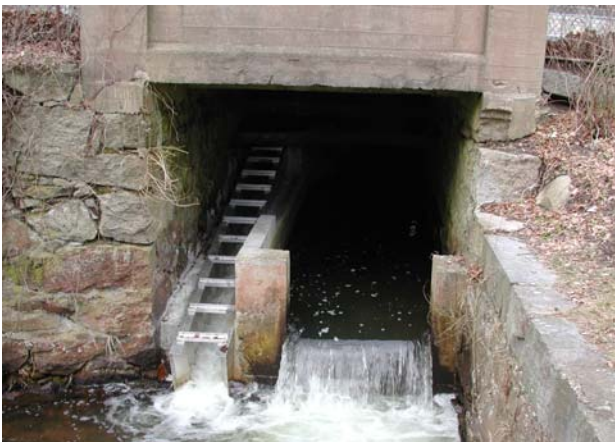
Newfield Street Fish Ladder
